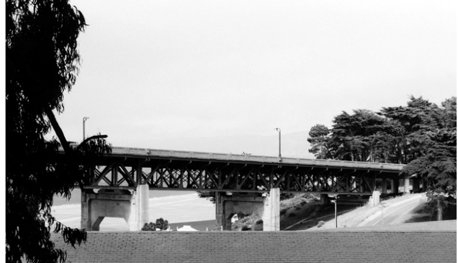
Doyle Drive viaduct structure
