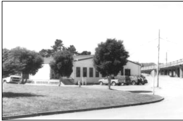
Exhibit 7-10 Main Post, Vicinity of Halleck Street, Building 230
