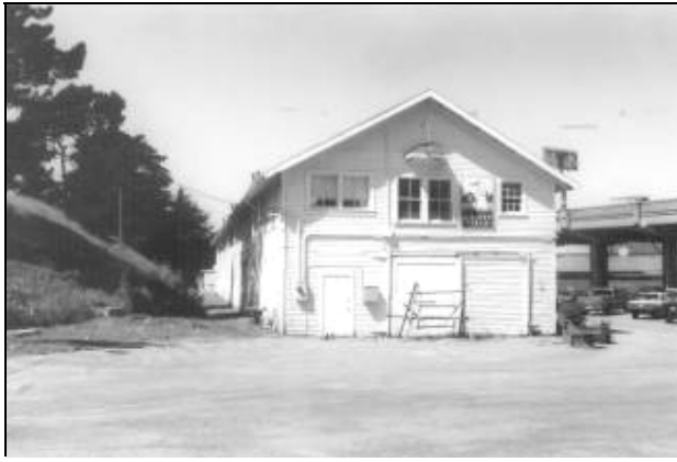
Exhibit 7-8 Main Post, Vicinity of Halleck Street, Building 204
