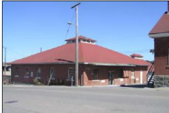
Exhibit 7-9 Main Post, Vicinity of Halleck Street, Building 228
