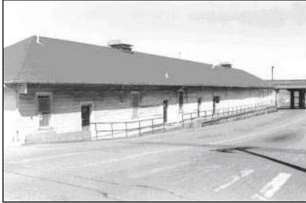
Exhibit 7-7 Main Post, Vicinity of Halleck Street, Building 201
