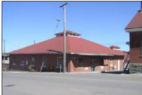
Exhibit 7-9 Main Post, Vicinity of Halleck Street, Building 228
