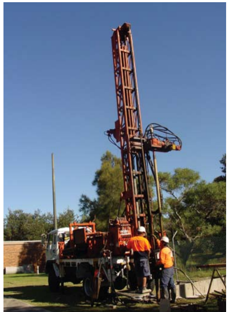
Truck mounted drill rig.
