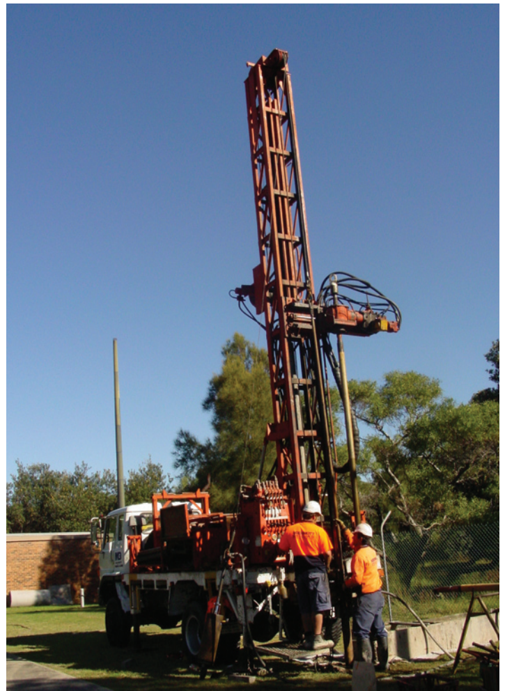
Truck-mounted drill rig.
