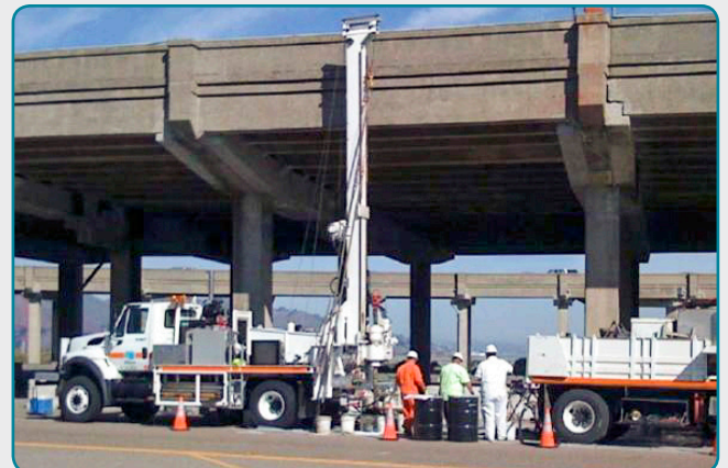
Truck mounted drill rig.
