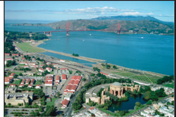
Existing Doyle Drive Aerial View
